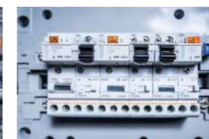
Electric Routine Inspection
