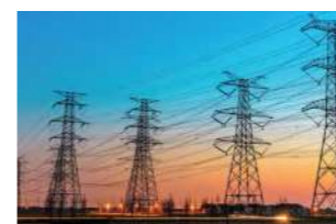
Electric Device Routine Inspection
