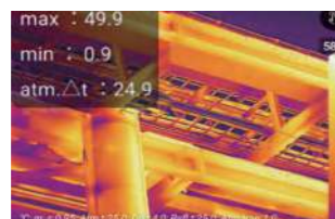
Chemical Operation and Maintenance
