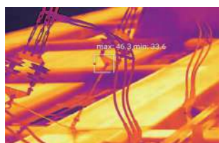
Electric Routine Inspection
