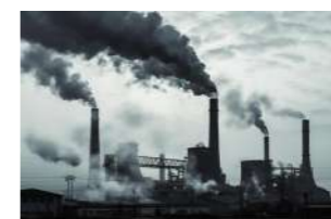
Emergency Response and Environmental Protection
