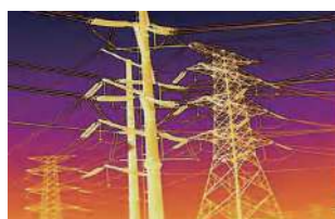
Electric Routine Inspection
