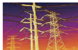
Electric Routine Inspection
