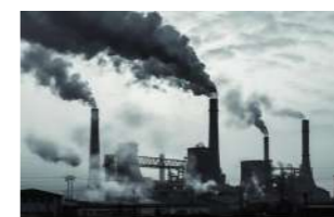
Emergency Response and Environmental Protection
