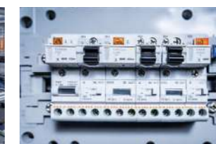
Electric Routine Inspection
