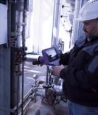
STEAM TRAP INSPECTION
